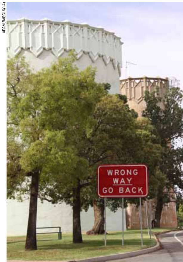
A SIGN of things to come in the Australian Rice Industry? Leeton's historic water towers, which are almost 100 years old, are reminders of how water availability and the town's fortunes are inextricably linked.
