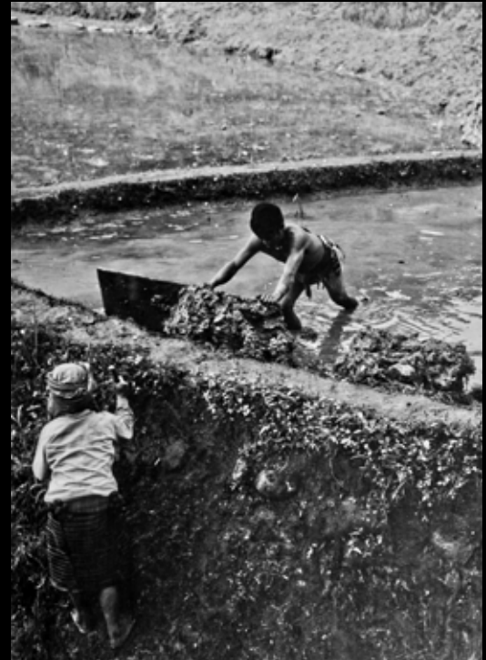
Terrace maintenance and dike repair are backbreaking work (1962).
