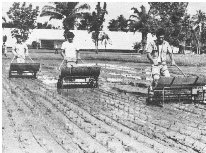
1. Rice transplanting machines being tested at IRRI.
